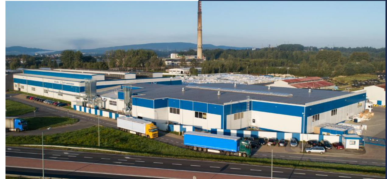
Sandwich Panel Factory, Gorlice
